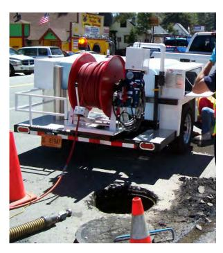
Purchasing our own video inspection equipment will allow the district to perform 100% of the collection system routine maintenance in house. The equipment consists of a remote-controlled crawler with a camera on the front and rear, video recording equipment, data logging and pipe condition software, pipe locating equipment and a support van.
