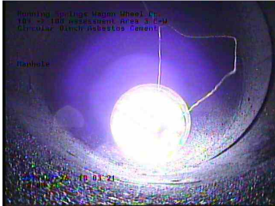
Assessment Area 3 E-W_0c2514d5-8ed5-49ee-a3c7-62334697154f_20190726_100558_371.jpg, 00:00:02, 0.00ft Manhole / 109
