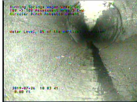
Assessment Area 3 E-W_0659b6af-67fb-4995-86d6-81194df0d4be_20190726_100619_141.jpg, 00:00:14, 0.00ft Water Level, 0% of the vertical dimension
