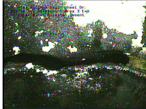
Assessment Area 3 E-W_4186542c-c536-411e-920d-0c9b34d38746_20190726_101126_586.jpg, 00:04:29, 49.85ft Joint Offset Medium
