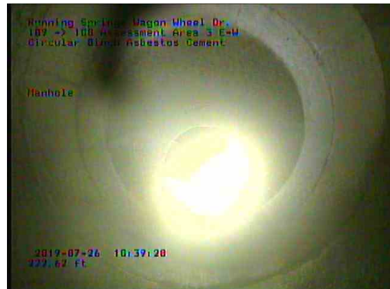
Assessment Area 3 E-W_2ff202fd-6caf-4149-92c3-25a48ffbde0d_20190726_104157_339.jpg, 00:19:00, 222.62ft Manhole / 108
