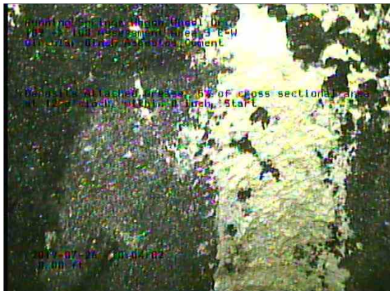
Assessment Area 3 E-W_3cb083e0-ee45-4325-951c-7954401242e6_20190726_100639_883.jpg, 00:00:24, 0.00ft Deposits Attached Grease, 5% of cross sectional area at 12 o'clock, within 8 inch, Start
