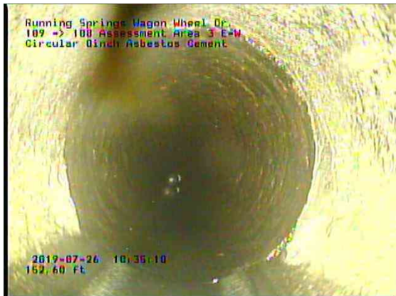
Assessment Area 3 E-W_0207bdcd-503b-4e1f-8e8e-fda9f1416e55_20190726_103755_955.jpg, 00:15:03, 153.02ft Material Change, Cast iron / 8"
